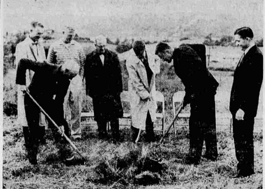
GROUND BREAKING ceremonies for the new Seventh-day Adventist School on NW Calkins Road were held Wednesday evening. Turning the first shovels of earth to mark the start of the long-planned project are, on left, Elder Ashley Emmer, center, Mayor Tom Garrison, and on right with shovel, Dr. Gerald Casebolt, chairman of the building committee. Looking on are, from left, Palmer Robson, school principal; Richard Callis, contractor; Elder J. R. Nelson, of Portland, director of elementary education for the Oregon Conference of the Adventist Church; and on far right, Dr. Duane Fletcher of the school board. (News-Review photo)
