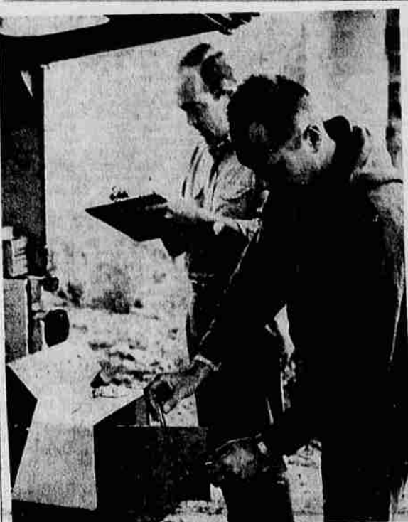
WATER TESTED — Chris Christanson, aquatic biologist for the state Game Commission, is shown at Roseburg Saturday testing the dye content in the South Umpqua to determine speed of travel of the river. The river at given points was checked at frequent intervals until peaks of concentration of the dye was determined. Then the crews moved on to the next testing point. Jotting down the reading is Pete Jeffs, hydraulic engineer for the U. S. Geological Survey. Heading the team was Dave Harris, USGS engineer. (News-Review photo)
