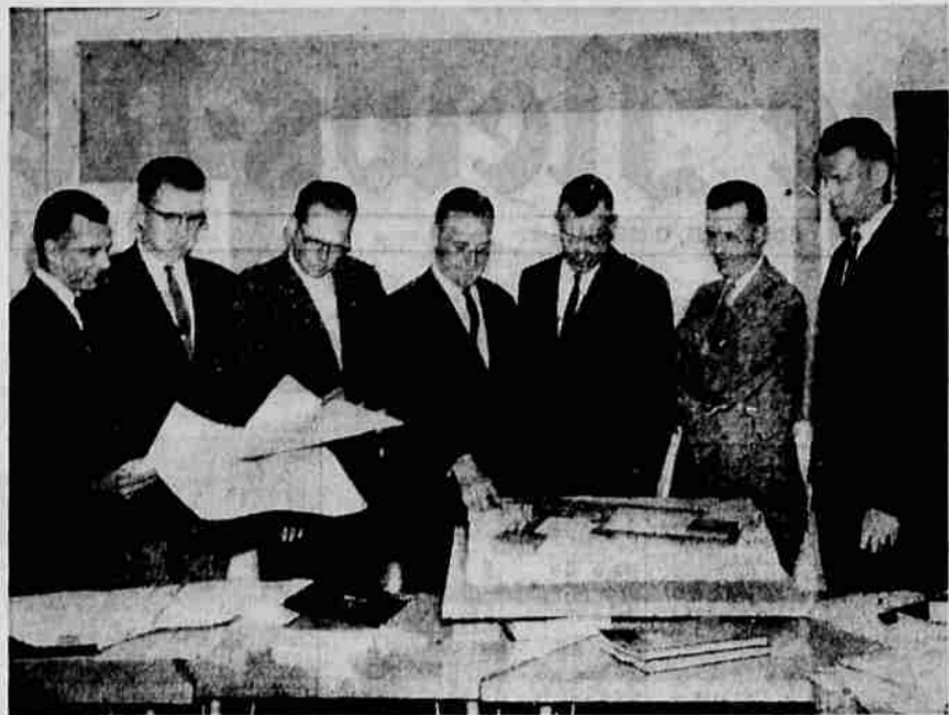
ROSEBURG SCHOOL BOARD members view a scale model and drawings of the proposed Winchester Elementary School at their regular meeting Wednesday night. After viewing the plans, the board gave architect John Briscoe the go-ahead to develop the basic plans shown in the scale model. Board members, left to right, are Dr. Verner Anderson, Art Lamka, Joe Dent, Ralph DeMoisy, Bert Young, chairman Dr. Nels Lindell, and Don Reed. (Bob Leber Photo)
