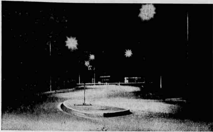
A NEW SYSTEM OF STREET LIGHTS is now in service from the railroad tracks on Washington Ave. to the Interstate Highway 5 underpass. Photo above shows some of the new lights as they illuminate a portion of W. Harvard Blvd. at nighttime. Picture looks southeast from the Roseburg High School curve. (News-Review Photo by Andy Fautheree)
