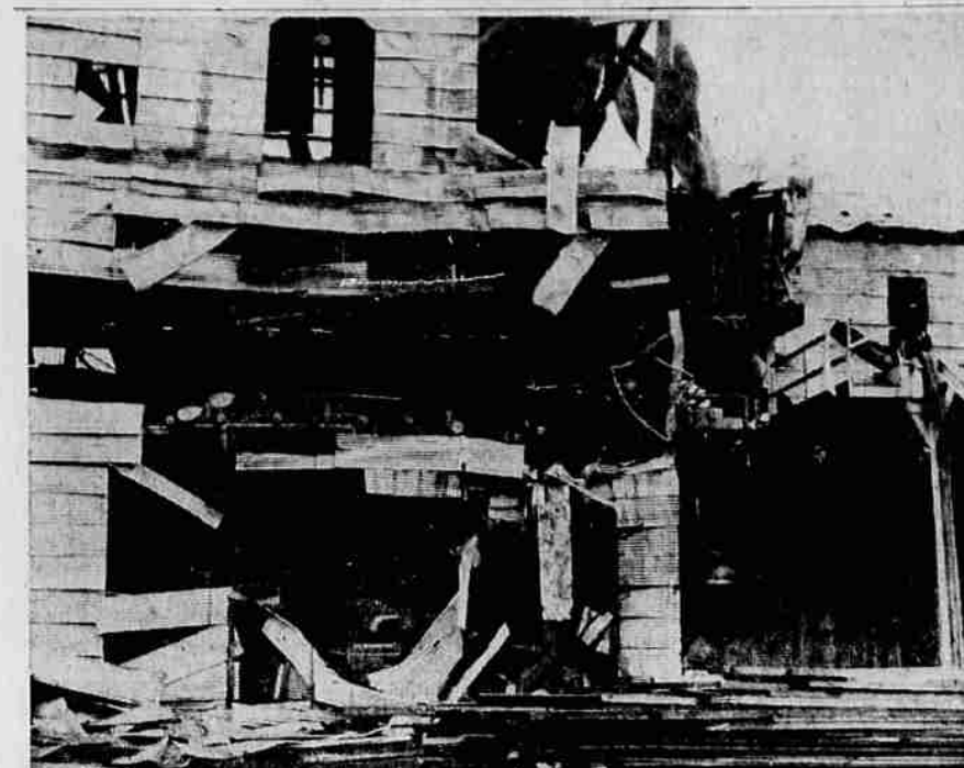
SAWMILL DESTROYED at the Martin Bros. Container and Timber Products Corp. at Oakland in a fire early Tuesday morning which officials of two fire departments said apparently started in this portion of the building. Oakland Fire Chief Fay Stearns and Roseburg Rural Fire Dept. Chief Cliff Thresher said indications were the fire was started when a compressor located in this part of the plant apparently blew up. (News-Review Photo)
