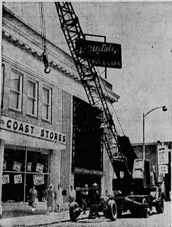
ANOTHER STEP in the long range plan to modernize the Equitable Savings & Loan building is the installation of a modern air-conditioning and heating system. Parts of the seven separate units were lifted to the roof of the building via a crane. The new system will replace the old steam heating methods. The entire building, including the Coast-To-Coast store will benefit. The long-range plan includes providing up-to-date modern office spaces also. Tozer's Heating and sheet metal is doing the work.
