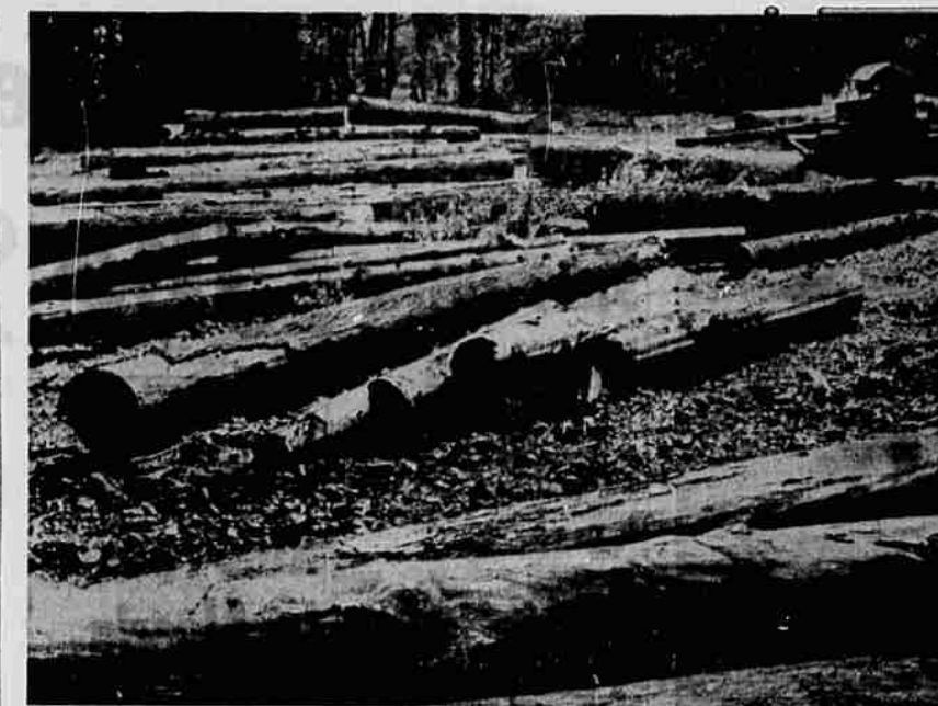
LOGS BEING CLEARED — Three accumulations of logs will soon be out of the streambed of Rock Creek, allowing Game Commission Fish Hatchery employees to breathe easier. Work is just being completed on the biggest jams to dispel much of the fear that high water might hurl the logs into the hatchery dam. Work is being done by Arley Fox of Lookingglass. The hatchery involves a quarter million dollar investment. See story page 1. (News-Review photo).
