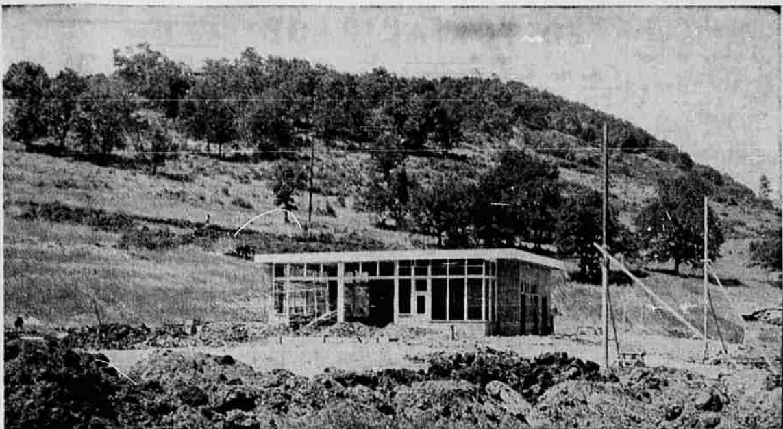
MAJOR CONSTRUCTION on the new Standard Oil Co. service station, as shown above, is nearing completion. The station is being built on the site off Highway 99 Freeway at the north turnoff leading to the Douglas County Fairgrounds. This is also the site of a proposed new motel, on which plans are still in the making. The station will serve as a first unit of the property location. Standard will lease the station to the Berman Corp., according to present announced plans. (Chris' Studio).
