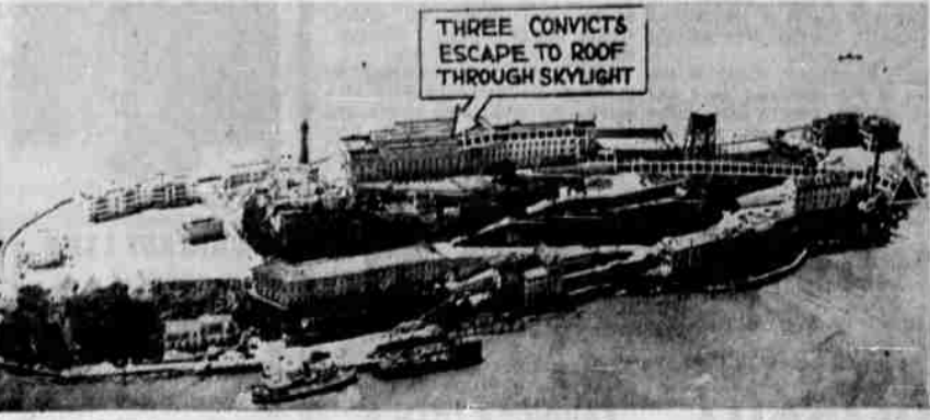
ESCAPE PATH — Prison officials at Alcatraz believe the three convicts who escaped Tuesday followed the path illustrated, fleeing from the roof of the building housing the cell blocks after climbing a pipe tunnel. The trio then is believed to have made its way to the northern end of the island, about 100 yards away, crossing two 12-foot fences before entering the waters of San Francisco Bay. (UPI Telephoto)
