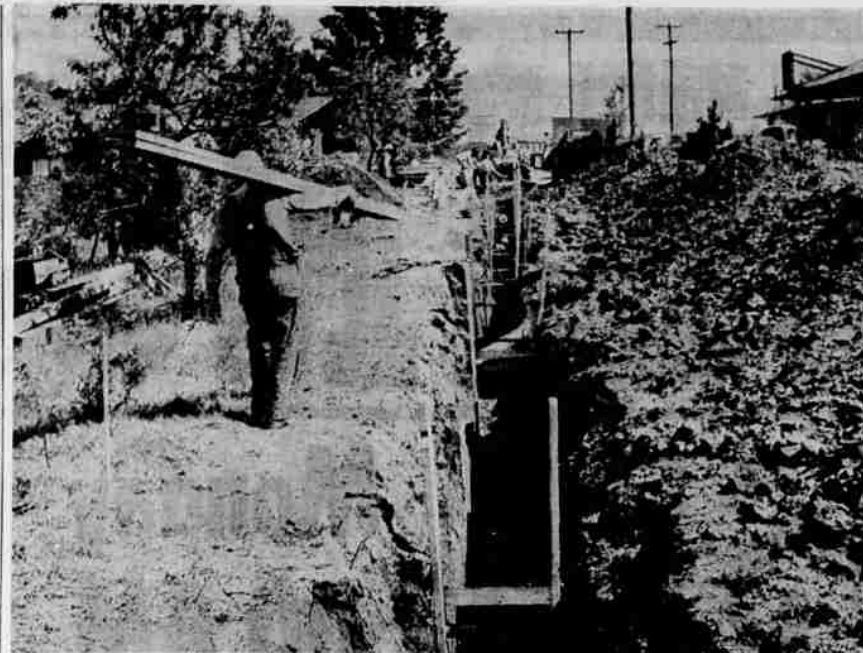
A SEWER SYSTEM for the Green Sanitary district has taken another step toward reality, with the start of construction for the laying of sewer mains pictured above. Selmor A. Hutchins has the contract at $400,052, with some variations. Completion date is Jan 17, although it is hoped the system may be in use sooner. The above work is started on the W. D. Myers property off Carns Rd., across from National Plywood plant. About 50,000 feet of pipe line will be laid. Work also has started on the stabilization pond for sewerage treatment (News-Review picture).
