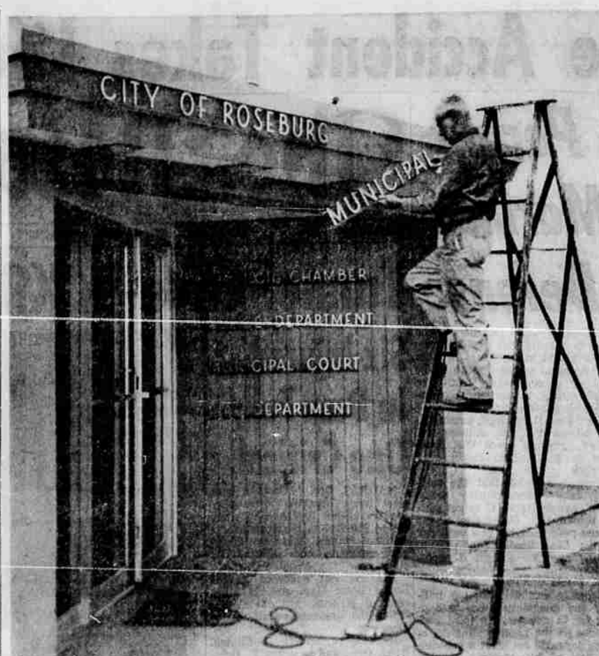
OFFICIAL NAME for Roseburg's newest municipal facility will be City of Roseburg Municipal Building. Above, Elmer Beckius, an employee in the street division of the Public Work Department, installs identifying letters on front of the building in preparation for dedication ceremonies tonight. The building, located at the corner of SE Rose St. and SE Lane Ave., houses the city's Council Chamber, Municipal Court, Police Department and Fire Department.
