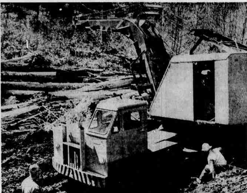
HOPES HIGH — Representatives of participating agencies watch with interest as work gets under way in stream clearance and spawning area restoration on Vincent Creek in western Douglas County. At top, a loader works on strewn logs, while below, a "cat" shoves some of the debris around. (Dawn Peseau photos)
