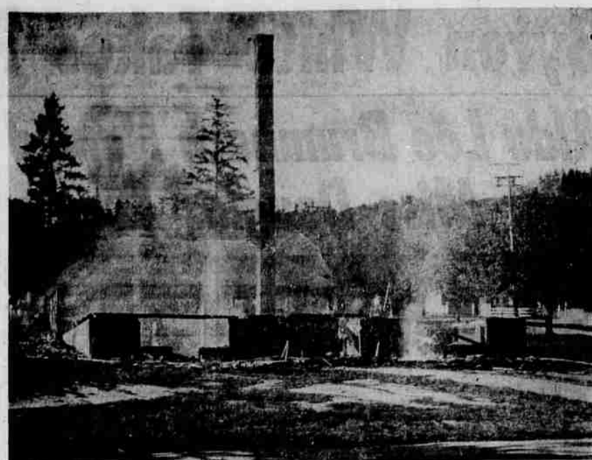
END OF AN ERA — The 51-year-old Sutherlin High School was reduced to a towering chimney and a smoldering foundation Sunday as the result of one of the most comprehensive fire-fighting training schools in the county's history. Firemen from all over the county, under the direction of state fire control officers, directed the training session under fire conditions. (News-Review photo)
