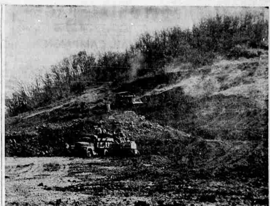
EARTH MOVERS eat deeply into the side of Reservoir Hill facing NE Stephens St., preparing a site for a new bowling alley. To be known as Indian Lanes, the alley will be owned and operated by D & D Bowling Inc., Richard Darby, excavator, has the contract to tear out part of the hillside to prepare for parking purposes and future building expansion, (Chris' Studio).
