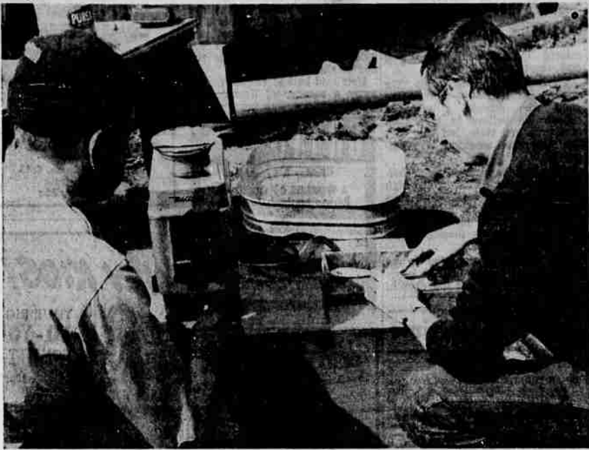
EXPENSIVE GADGET — Bob Garrison, Game Commission aquatic biologist, and Andre Coche of Belgium, doing graduate fisheries studies, are shown here using a new electric fish weighing scale. The machine costs $500 and gives an instant reading on the weight of the live and wriggling fish. Sample fish from those gathered at the Whistler's Bend natural rearing pond this weekend were weighed in this manner.
