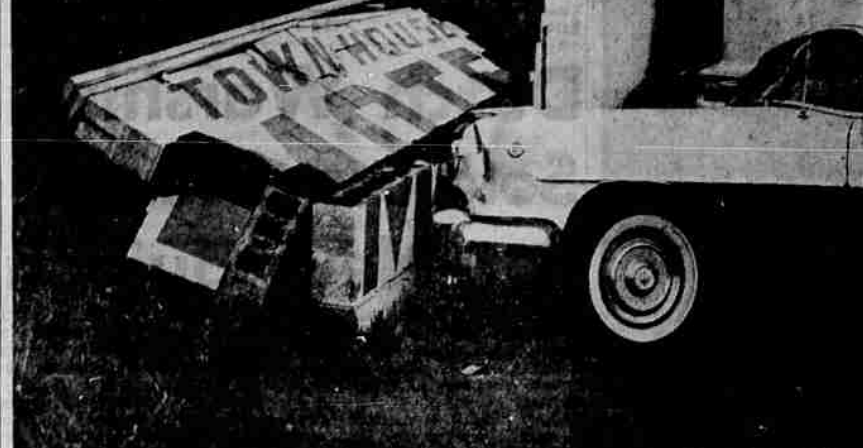
WHOOPS — The car above, registered to Herb Pomeroy of Roseburg, went out of control and turned into a battering ram this week. It slammed into the cinderblock retaining wall at Town House Motel on NE Stephens St. The impact not only ruined the wall, but raised havoc with the motel's sign.
