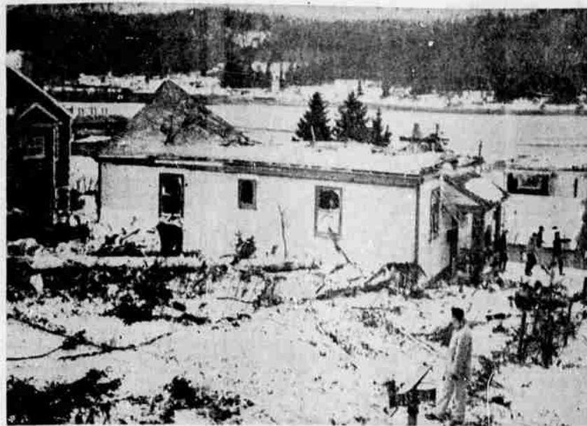
12 HOMES DAMAGED — The aftermath of an avalanche is shown here when 12 homes in a residential district of Juneau, Alaska, were damaged by a huge snow slide which roared down 3,500 foot Mt. Juneau in the pre-dawn darkness Thursday. The snow slide sheared off about 200 trees in a 200-foot swath before it crashed into the homes. Apparently the only injury was a housewife who suffered a leg cut. (See story, page 2, second section). (UPI Telephoto).
