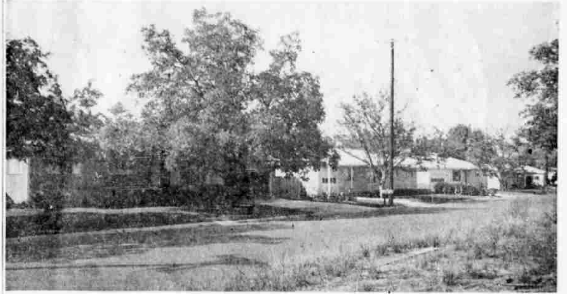
OCCUPIED THIS SPRING — Most of the homes pictured above were constructed this spring by Ivan Edwards in the Quintus Park Addition, north of W. Harvard Ave., and have been occupied since completion. There are several
