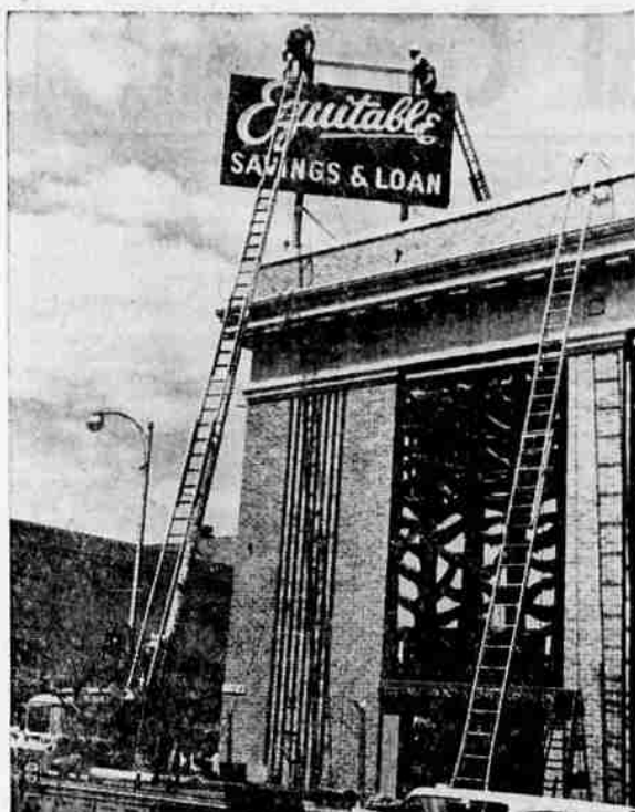
BUILDING ALMOST READY. —The grand opening of the Equitable Savings and Loan Association headquarters in Roseburg is scheduled next week. Meanwhile the company has just finished installing the new sign atop the two-story structure. (News-Review Photo).
