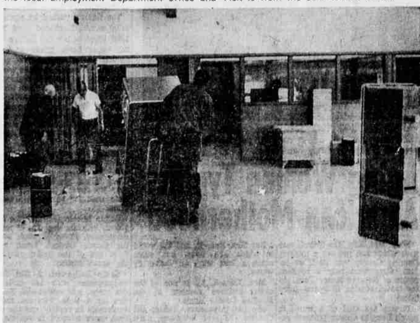
MOVING IN to the new Employment Department offices was carried out Thursday and Friday, as the recently-completed building was made ready to be open to the public Monday morning. It was designed by Eugene architect James Keefe and Constructed by Todd Building Co. of Roseburg.
