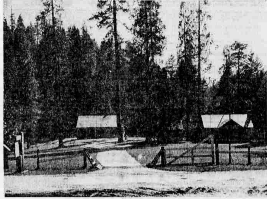
DEVILS' FLAT GUARD STATION, located near the end of the county controlled portion of the Upper Cow Creek Road and the beginning of the portion controlled by the Forest Service, presents a beautiful sight to travelers of the road with its well kept, spacious grounds. The Forest Service keeps several picnic tables available here for the public's use.
