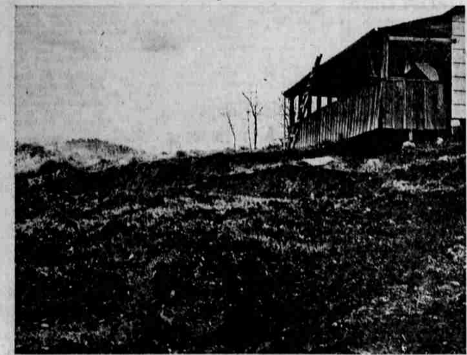
SLIPPING OF SOFT EARTH on the hillside in the south part of town is threatening the above pictured residence of William P. Donnelly, 1335 SE Marsters St. Heavy rains during the winter months have loosened the earth, causing it to slide down onto the street. The northwest corner of the porch support is now exposed. The soft earth started giving way after part of the slope was cleared of brush and terraced. (News-Review Photo)
