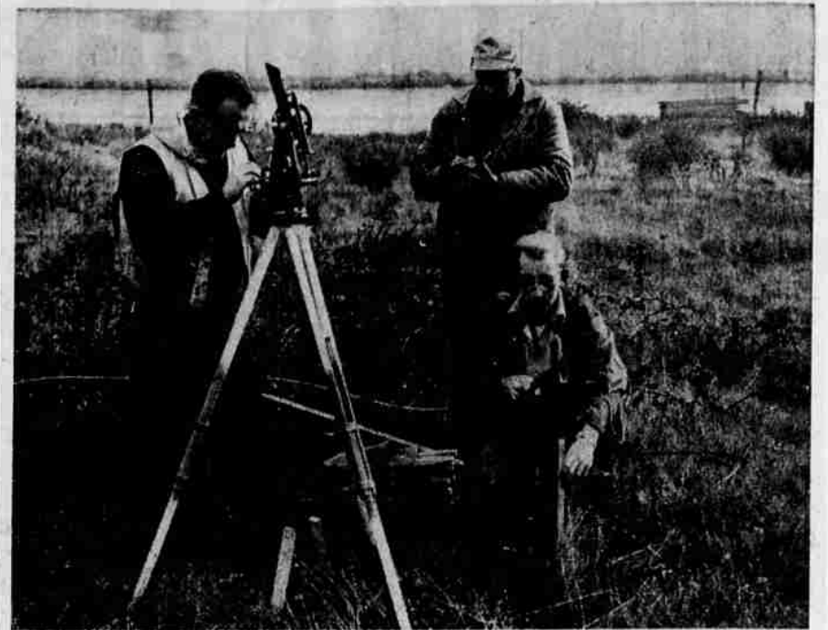
STAKING OUT A NEW ROAD , a county surveying gang is beginning preliminary locating near Riddle. The road is to be the new Riddle by-pass stretch. From left are shown Don Garrett, 450 W. Cochran Ln., transitman; Ron Curry, 3260 Broad St., chairman; and, kneeling, Garry Heichel, 327 SE Lane St., head chairman. (News-Review Staff Photo)
