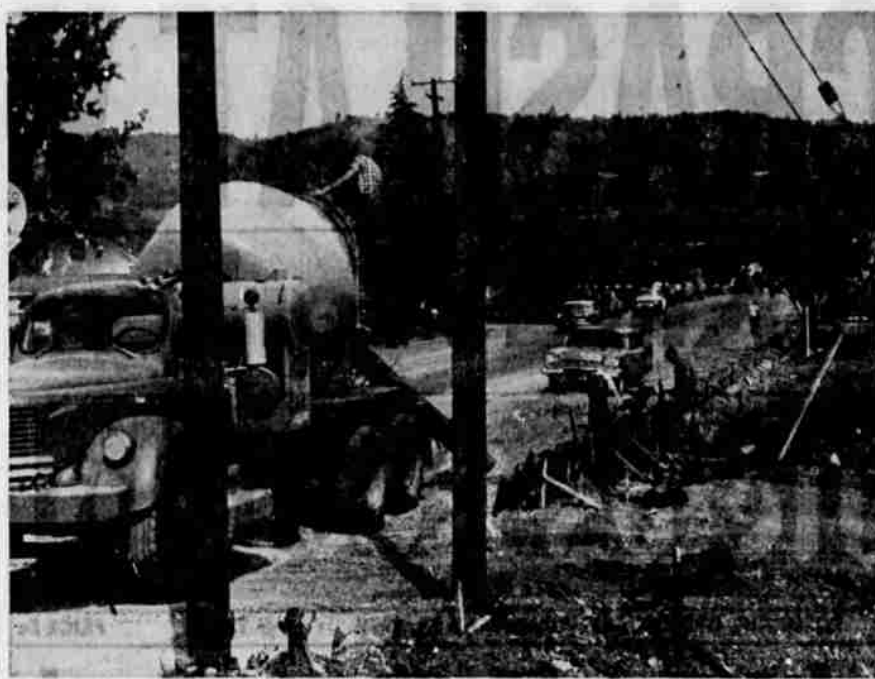
GARDEN VALLEY BLVD. construction moved forward this week as the heavily traveled Roseburg traffic artery is widened to four lanes. Currently Inter-City Sand & Gravel Co., Inc., of Eugene, is putting in curbs and gutters. Work shown here is on the south side of the road looking east toward the city. (Paul Jenkins)
