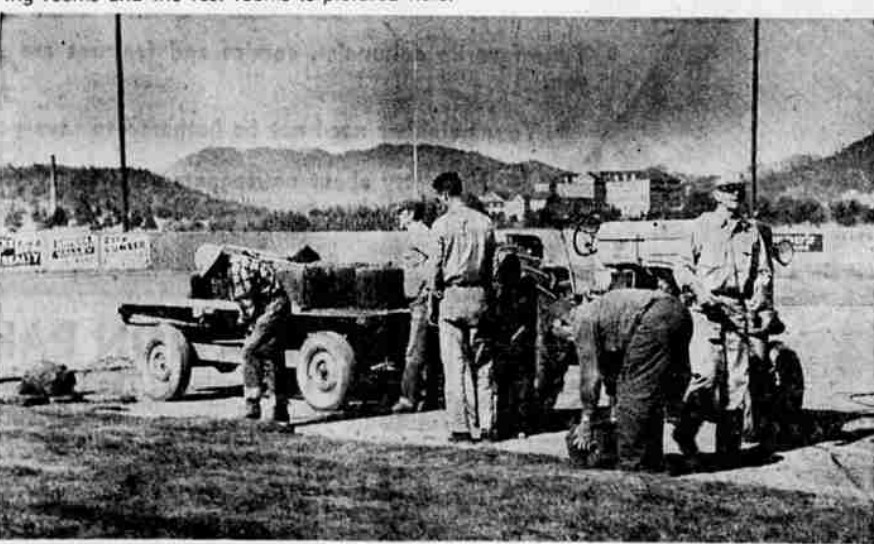
ANOTHER LOAD — Workmen begin to place another load of strips of turf in place on the Legion Field infield. The strips of sodded turf are removed from the Veterans Administration grounds and transported to the ball park in rolls. Rudie Ritzman, former city councilman instrumental in the completion of the field, is on the far right. The new turf is expected to be installed by this weekend.
