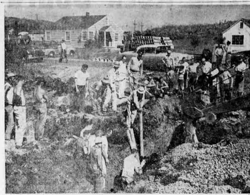
TENSE MOMENTS are experienced by onlookers and rescuers as Clarence L. Stone, 39, of Glida is pulled from an excavation project cave-in. Stone was trapped when dirt and shale caved-in on him while he was working on a sewer construction project. The Salem Sand and Gravel Co. employee was rushed to Mercy Hospital after he was freed from the hole.
