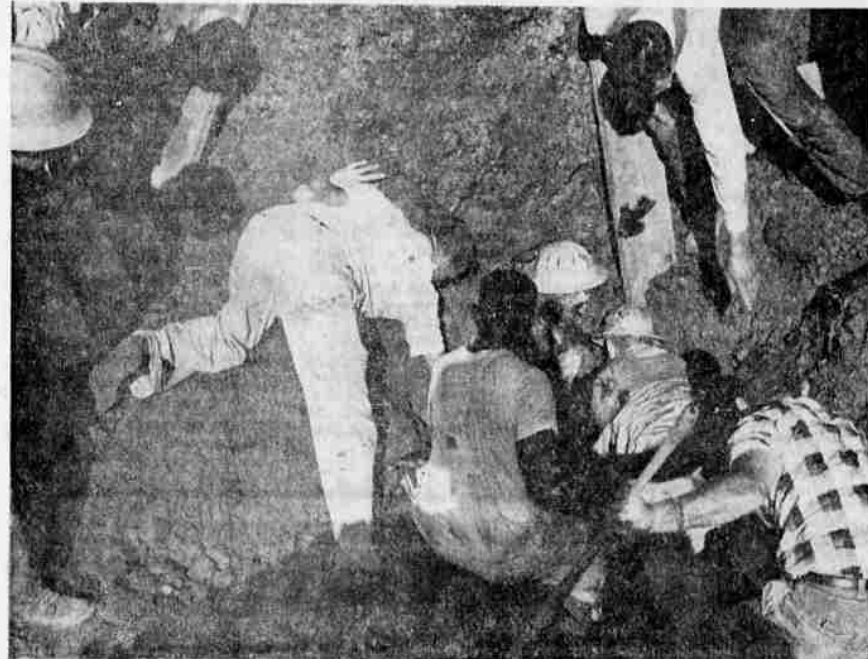
TRAPPED — Roseburg firemen and employees of Salem Sand and Gravel Co. work to free 39-year-old Clarence L. Stone of Glida who was trapped in a cave-in Tuesday afternoon. The accident happened on a sewer construction project in west Roseburg. (Paul Jenkins)
