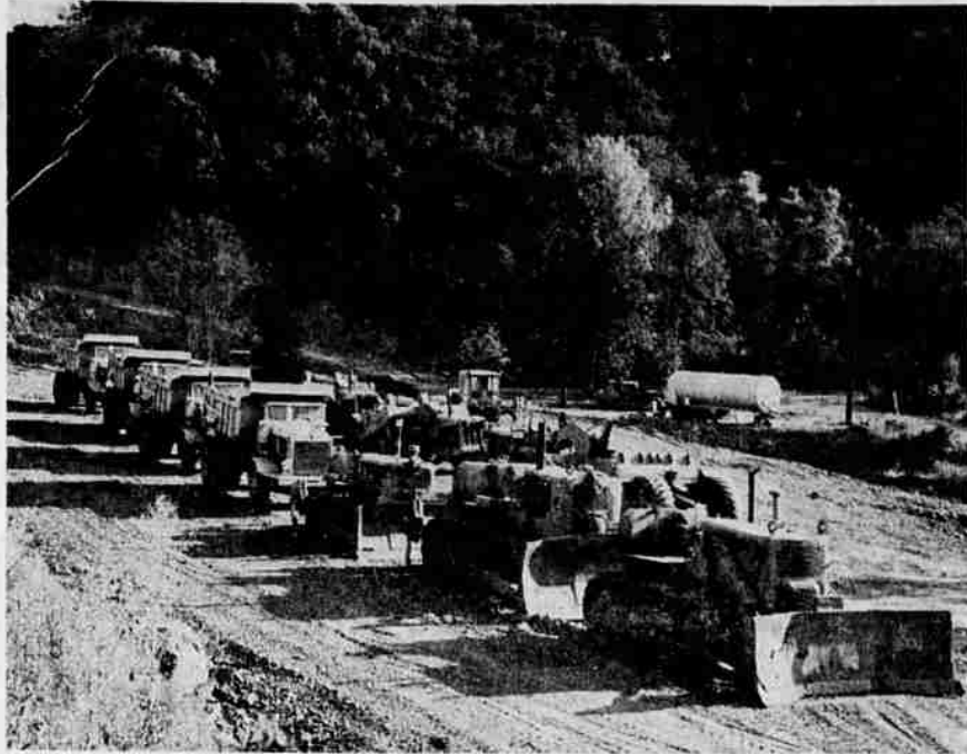
HEAVY EQUIPMENT of O'Neill Construction Co. rests at the foot of Roberts Mountain where it was lined up when heavy construction was halted by a strike-lockout. When the green light comes on, the machines will be put back to the job of joining two four-lane sections of Highway 99.
