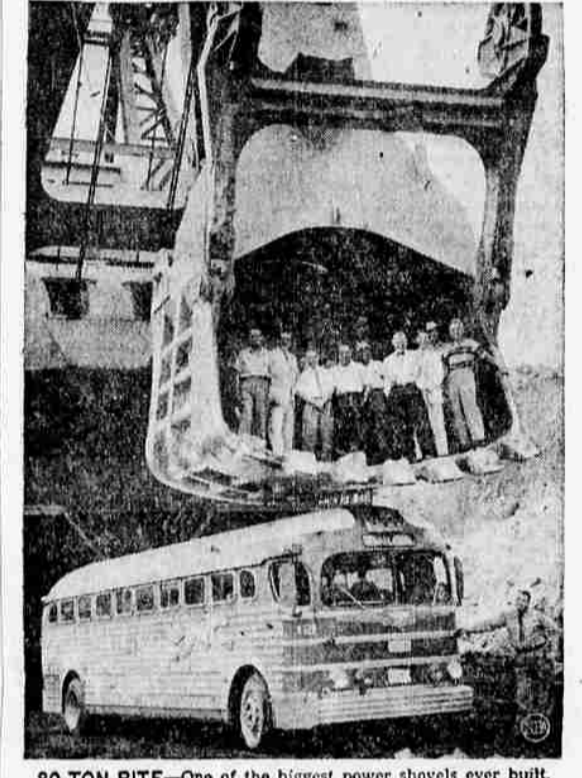
80-TON BITE —One of the biggest power shovels ever built, the River Queen, was recently put in operation near Central City in the western Kentucky coal field. The big shovel is capable of biting out more than 80 tons of rock and earth at one time. Note size of scoop as compared with bus below and men standing in its mouth.
