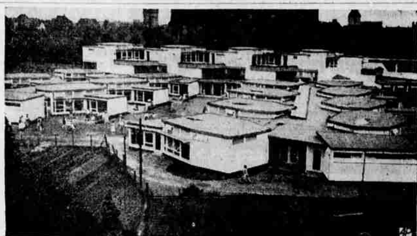
SCHOOL MAZE — This is a view of a new high school for girls in Luenen, Germany. What looks like a maze of geometric shapes is a series of wings with classrooms in hexagonal shape. Rooms are distinguished inside by different colors and furniture.
