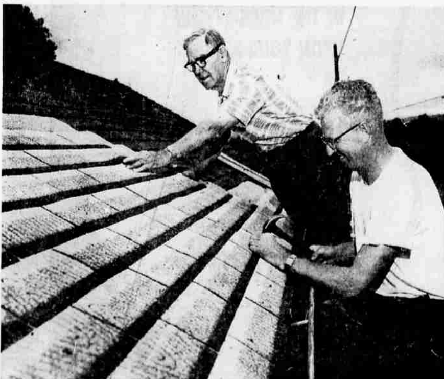
ANOTHER NEW ROOF BY WARDS — Glen Wellman of 1086 N. E. Walnut Street is shown inspecting his new roof installed by Leo Kawalewski, local roofing installer. They are reroofing Glen's home with WARDS new 3-tab Shingles with a 10 year guarantee against defective material or workmanship. Phone ORchard 3-5553 for your FREE estimate a WARDS Building Supply Department.
