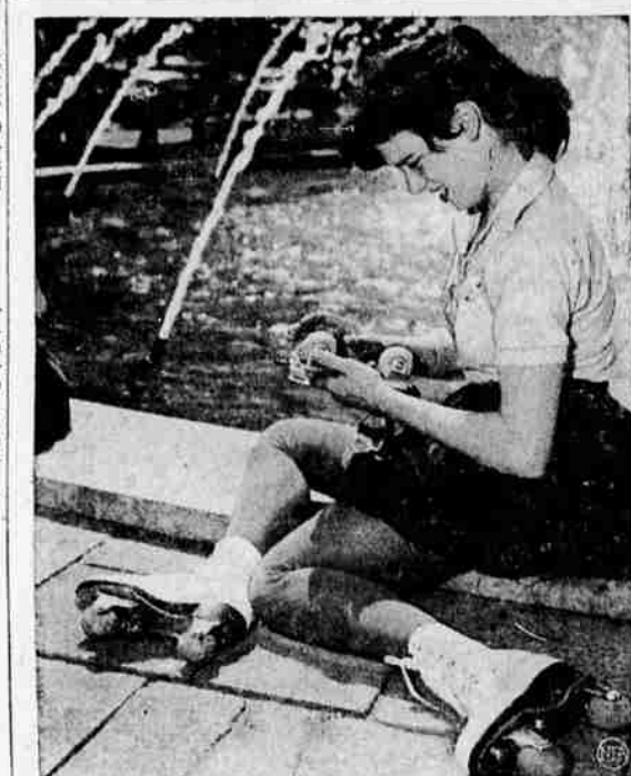
TWO-WHEELING — This young lady seems to be amused as she examines the latest in roller skates. The new skates, manufactured in West Baden, Germany, feature two hard rubber balls in place of the conventional four wooden or steel rollers. The manufacturer claims the skates are safer because they can't slip sideways. They are also much quieter than the standard skates.
