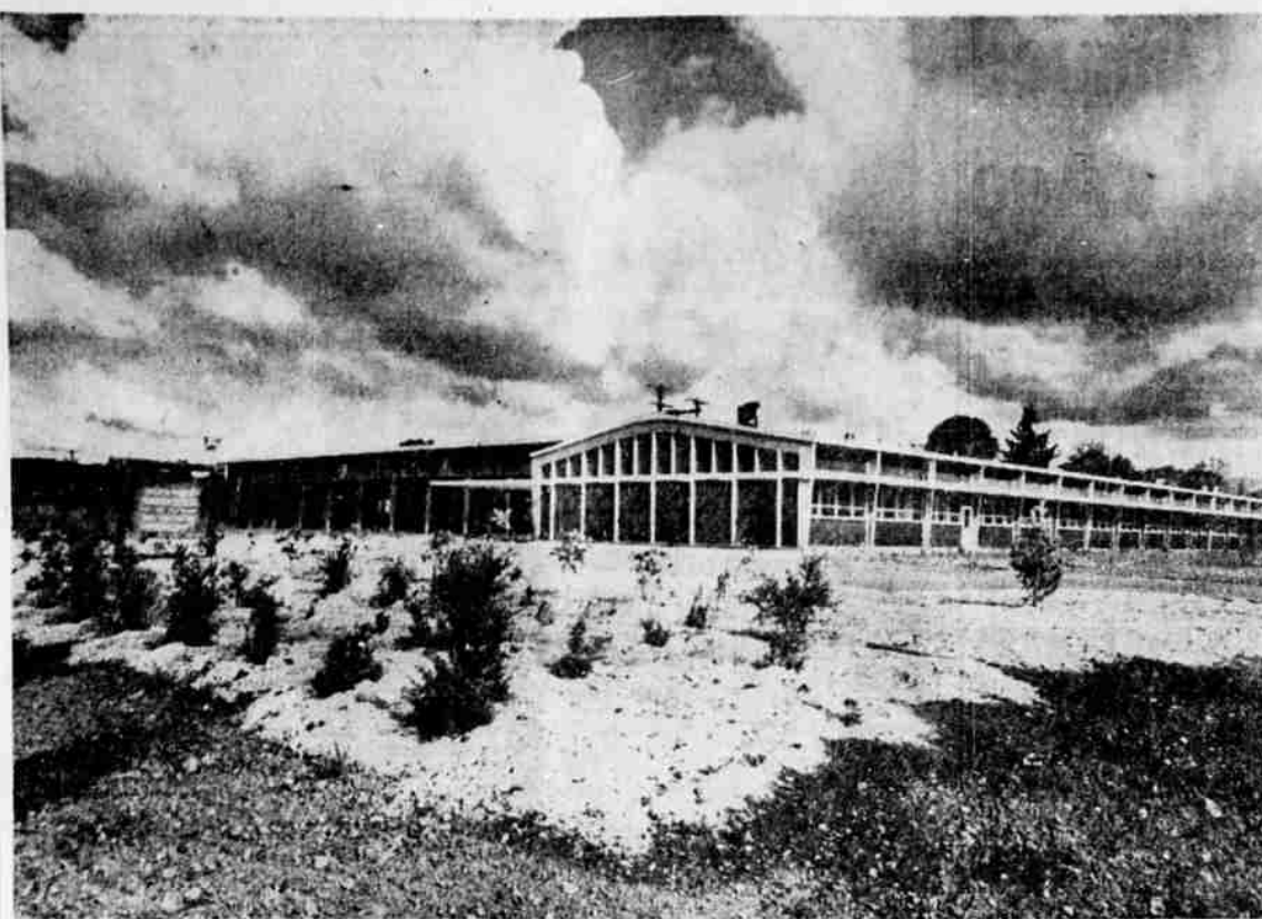
RESEARCH CENTER — The Oregon Forest Products Research Center is now in a new home, above. The expanded and improved facilities form a monument to the necessity and importance of forest research. Fittingly, the
