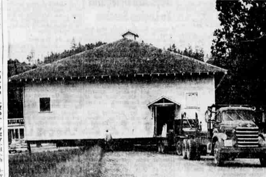
MOVING DAY — A 110 by 92-foot Glide School gymnasium was moved Friday from school property to a lot leased by the Glide Community Club on the North Umpqua Highway. The school district donated the building. While the structure was being moved the highway was closed to traffic and vehicles were routed over the old highway. Ahre and Richmond, a Eugene firm, had the moving contract. About 3 p.m. Friday dollies under the front of the gymnasium mired in mud at the new location and the movers were trying to raise the building today. (Paul Jenkins)
