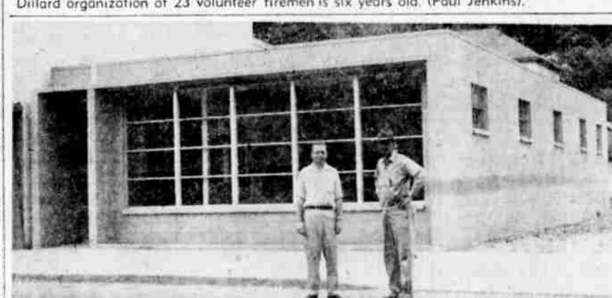
NEW DRAIN POST OFFICE is nearly finished and probably will be occupied about June 1. Installation of mail boxes and some finish work are all that remain to complete the building. Postmaster Harry Cool Jr. and contractor and building owner Steve Ferche, Roseburg, are in front of the building. Ferche will lease the building to the U. S. Post Office Department for 10 years, with two five-year option periods. (Drain Enterprise photo)
