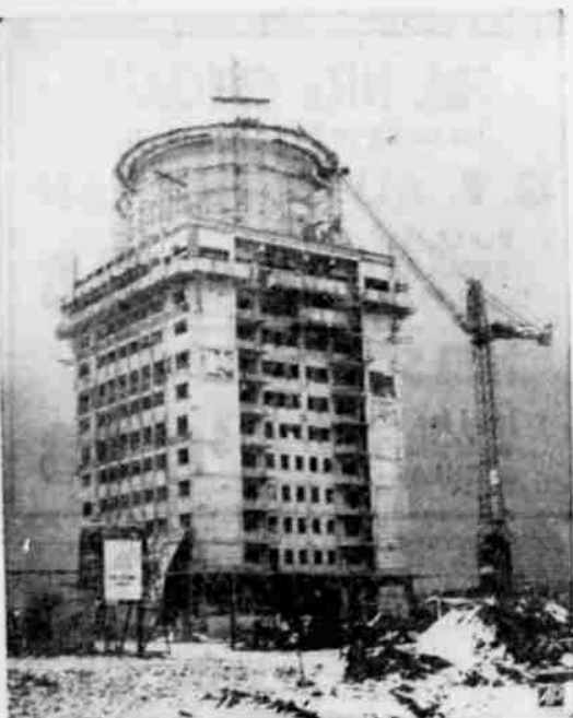
DUAL PURPOSE —Frame of this 12-story apartment house in Velbert, Germany, is built around a water tower. Project disguises tower and conserves valuable ground space.
