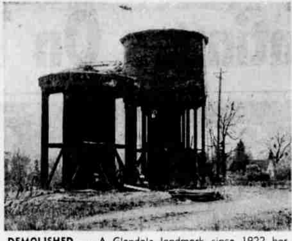
DEMOLISHED — A Glendale landmark since 1922 has been demolished. Southern Pacific crews recently completed dismantling two water towers which were used when Glendale was a busy railroad center and trains needed water. The towers were not needed after diesel engines took the place of steam. At one time the city considered purchasing the tanks for water storage for fire protection.
