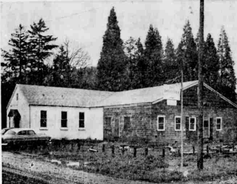
NEW EDUCATIONAL UNIT to be dedicated Sunday at the First Baptist Church in Drain is shown above. The $10,000 structure was built primarily through the donated efforts of church members.
