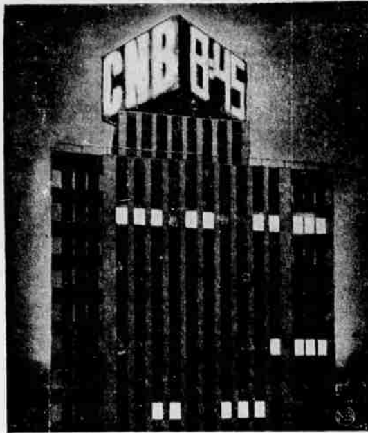
CLOCK IN THE CLOUDS —The world's largest super-accurate clock was recently put into operation atop the 30-story Continental National Bank Building in Fort Worth, Tex. The clock makes one complete revolution every minute and flashes the time minute by minute in giant illuminated numerals over two stories tall. It can be read day or night at distances of three miles or more. Accuracy is controlled within 1/20th of a second by a short wave signal from the National Bureau of Standards Transmitter at Beltsville, Md.
