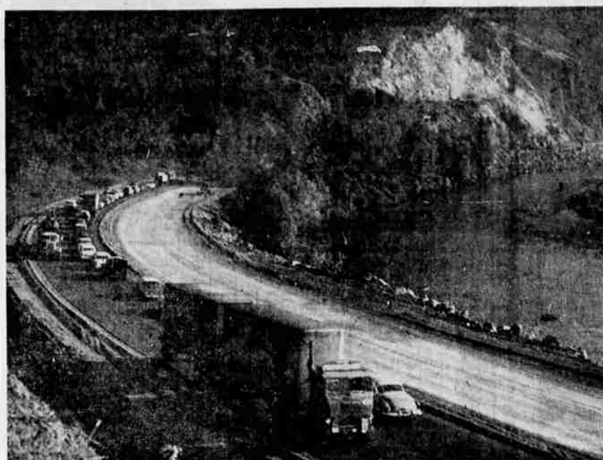
ONE-WAY TRAFFIC AHEAD — Traffic on Highway 99 is now moving over a temporary surface on a new grade along Umpqua Bend south of Myrtle Creek. Construction, however, limits traffic to one way part of the distance on the new grade, and the contractor has a pilot car to lead motorists through the construction area, which can be seen in the right background. (Staff photo)
