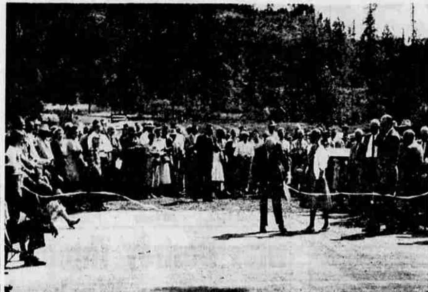
BRIDGE OPENED — Floyd C. Frear, county road engineer for 36 years before his retirement in May 1956, snips the ribbon that opens the North Umpqua Bridge named for him. Watching closely is Jean Lundstrom, daughter of John Lundstrom (tall man at right), representative of West Coast Steel Works, the builder. The present Douglas County Court and former court members attended, and are standing at far right with Lundstrom. They include: Commissioner Huron Clough, Judge V.T. Jackson, Commissioner Frank Ashley (face hidden behind Lundstrom), ex-Judge Carl C. Hill (wearing hat) and ex-Commissioner E. R. Metzger. Man farthest on right is unidentified. A crowd of several hundred attended. Jackson and Hill spoke. (Paul Jenkins)
