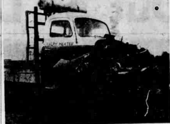
TRUCKS COLLIDE—Ralph Clyde Heater, 43, Rt. 4 Box 525, Roseburg, received minor injuries Wednesday morning when his unloaded short logger collided with another truck driven by Alfred Louis Denton, 33, of 2028 NE Airport Rd., Roseburg, at the junction of the Kent Creek, Rice Creek and Dillard-Brockway roads just south of Dillard. Both trucks were heavily damaged, state police said. (Staff photo.)
