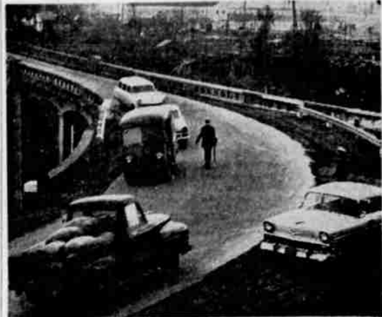
ROADBLOCK—State police and deputy sheriffs ringed the Tri-City area with roadblocks Monday afternoon. This one was at the bridge at Myrtle Creek during the search for gunman who stole a police car. (Paul Jenkins).
