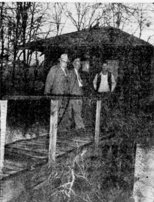
PUMP STATION for the mineral springs on the proposed hospital site is surveyed by three officers of the children's hospital and rehabilitation site at Boswell Springs. They are left to right, E. G. High, Roseburg, executive director; Dr. Harrison Folk, resident chiropractor; Richard A. Duncan, Drain, president of the board of directors.
