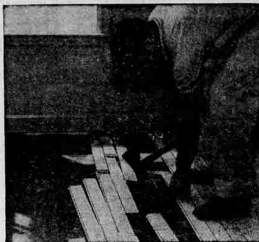
MOST OAK FLOORING USED NOWADAYS is tongued-and-grooved at the ends and sides for snug, easy joining. In installation, the flooring is toenailed. The richness of polished oak helps set decorative themes for any decor—modern or traditional; its neutral color blends with any color scheme.
