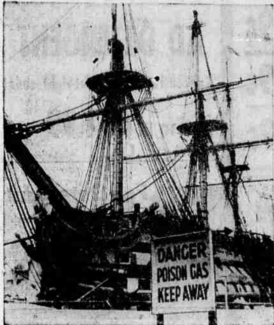
GAS WARFARE —A modern military weapon comes to the aid of an ancient war vessel in Portsmouth, England. Lord Nelson's historic flagship, H.M.S. Victory, is pumped full of poison gas and her hull sealed off to kill death-watch beetles eating at her timbers. Fumigation by methyl bromide gas is carried out periodically.
