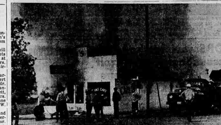
FIRE AT RIDDLE Wednesday caused between $4,000 and $5,000 damage when it attacked Lynn's Cafe and an apartment. Two newspaper carriers turned in the fire alarm. Fire Chief Don Holcomb said it was believed the fire started from a burner beneath a gas heater. The building was owned by Mrs. Cora Cloud. Living in the apartment were Mr. and Mrs. Lynn Cloud. (Ken Hunt).
