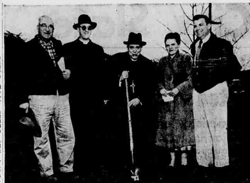
NEW SUTHERLIN CHURCH —Ground breaking ceremony for the Church of the Holy Spirit was held this month in Sutherlin. Construction on church will start immediately. Ceremony brought honored guest, Bishop Benjamin D. Dagwell, Portland, Diocese of Oregon, center. Church is second new Episcopal church started in county in past two years. From left: William Mordin, junior warden; Father Alfred S. Tyson, St. George's Episcopal Church, Roseburg; Bishop Dagwell; Mrs. Fred Dietrich, guild president; Russell Cooper, senior warden. (Photo Lab.)
