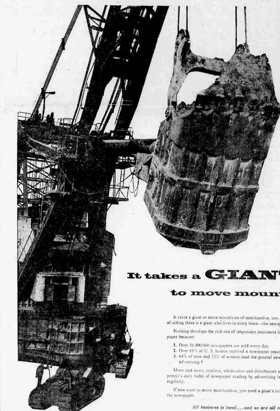
Giant shipping shovel built by Bucyrus-Erie for Union Hill Coal Co., New Lexington, Ohio. Dipper scoops up 45 cubic yards at a gulp.
