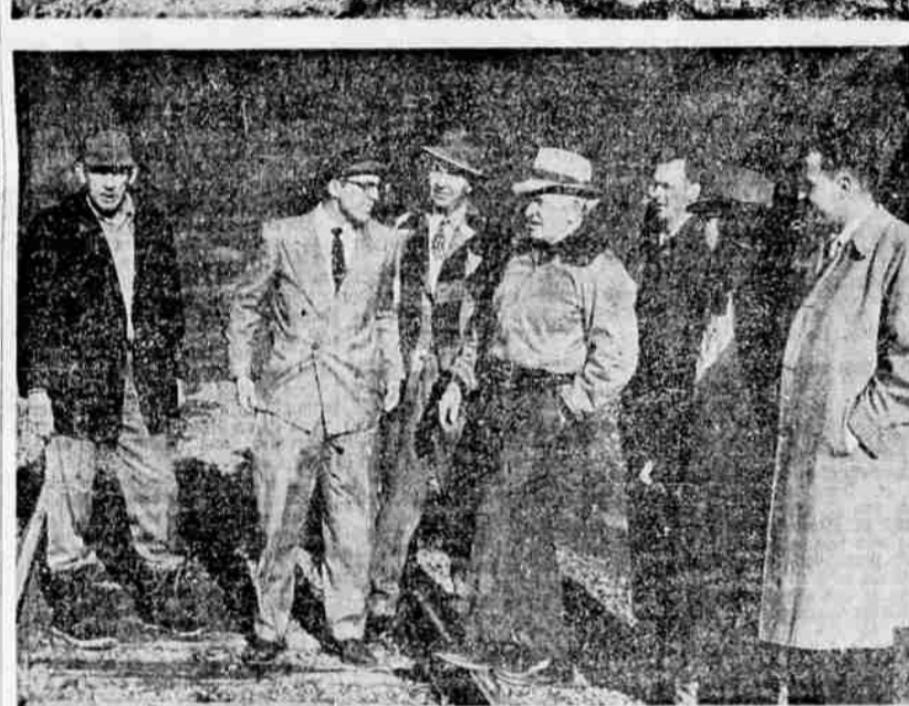
POINT IN QUESTION—Charges that Southern Pacific Co. is dumping slide material into the South Umpqua River north of Dillard were surveyed Monday by railroad officials, citizens and observers. (Top) Three slides in this area are trouble spots. River curves wide here. Winston Falk says current has altered causing flood damage. (Middle) SP suffered slide damage. Communication poles were knocked asunder. Ben Irving observes. (Bottom) Friendly protagonists in slide survey were J. N. Cetinich, SP official, second from left, and Gen. Curtis T. Beecher, fourth from left. Others from left: Fred Gustafson, State Engineer's office; Cetinich; O. D. Young, SP; Beecher; Arnold Severson, State Highway Dept.; Fred Odgers, SP; and Jack Neby, SP. (Paul Jenkins).
