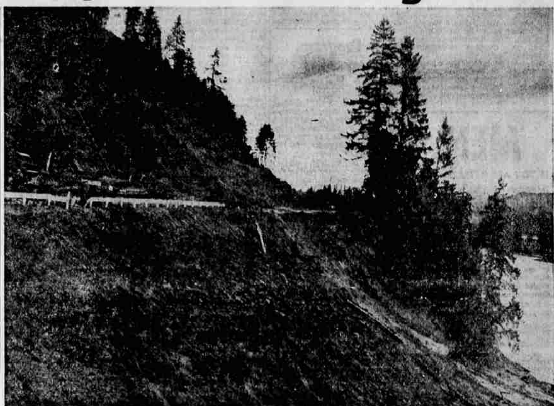
HUGE SLIDE about two miles east of Reedsport blocks vital highway link between coastal and inland points. Highway blockage has brought ferry and train into use.
